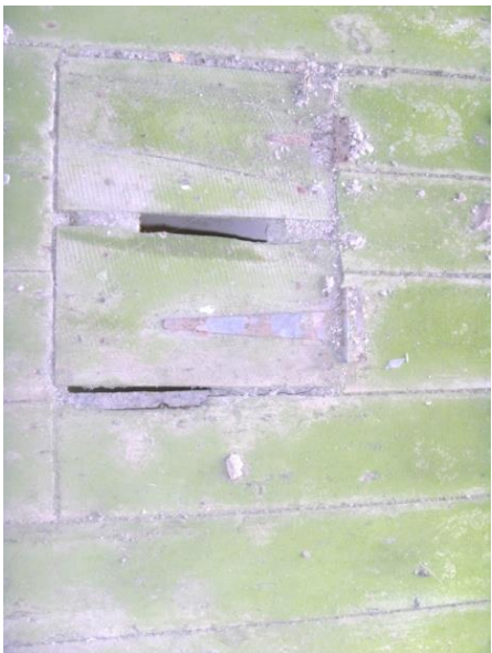
A (cat) flap in the upper floor of loft shows metal strips between the boarding.
