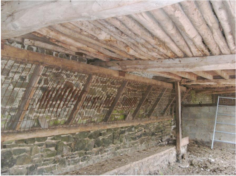
Feeding racks beneath the fir poles in the linhay
