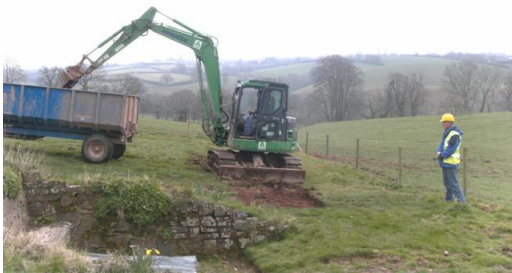
Chris Preece supervising the mechanical digger opening T4 in the garden
