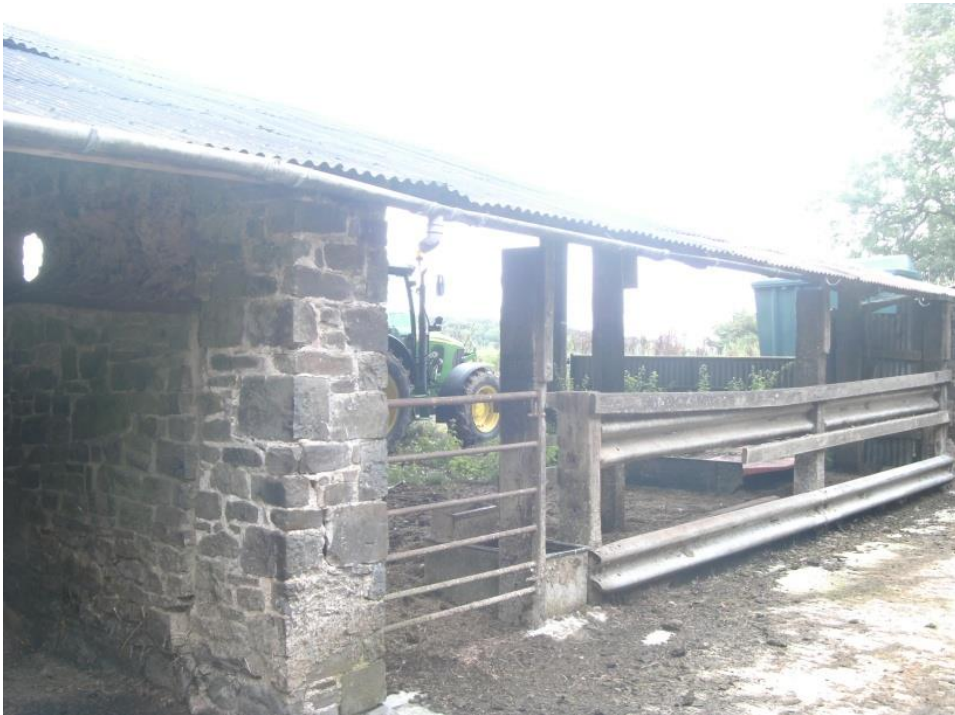
A modern extension to the old linhay
