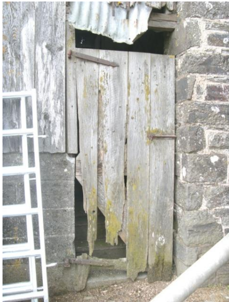
Entrance door to stairs to upper floor of the engine house loft
