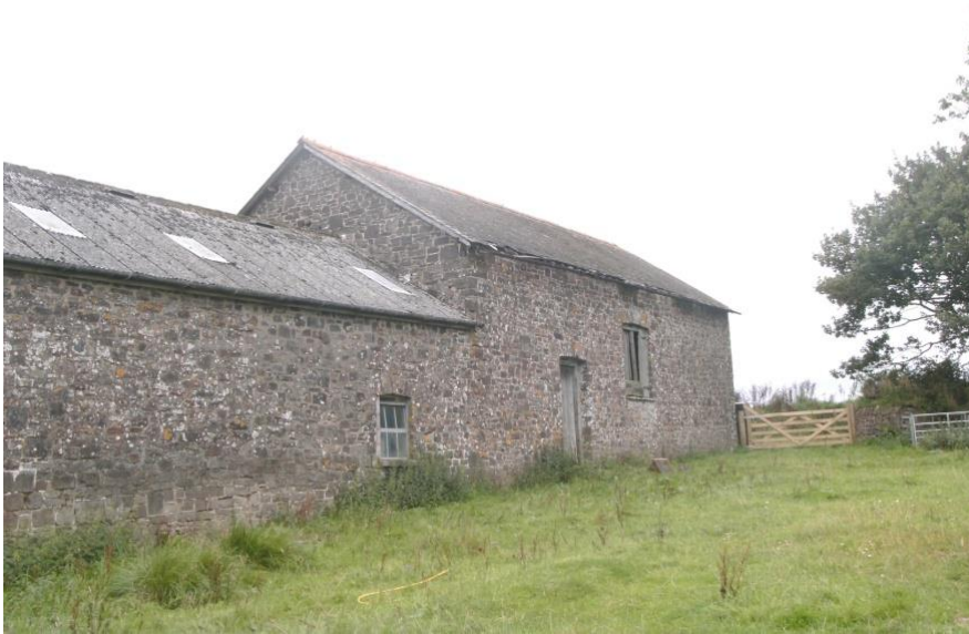
Eastern elevation of granary and barn, north-south
