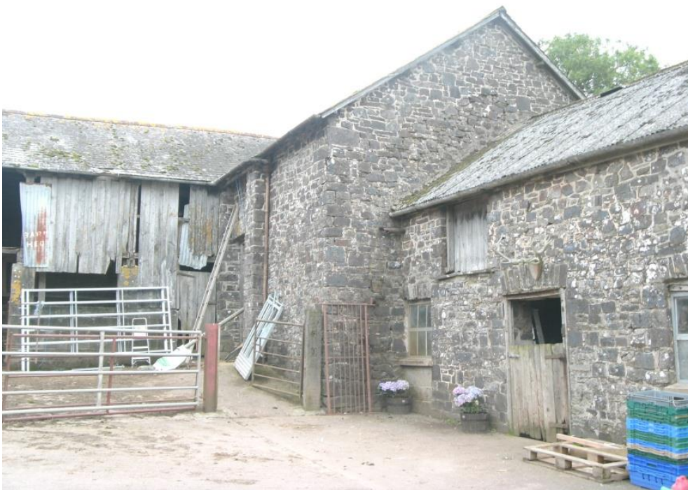
North-east corner of range of buildings; shippen, granary and loft in need of repair
