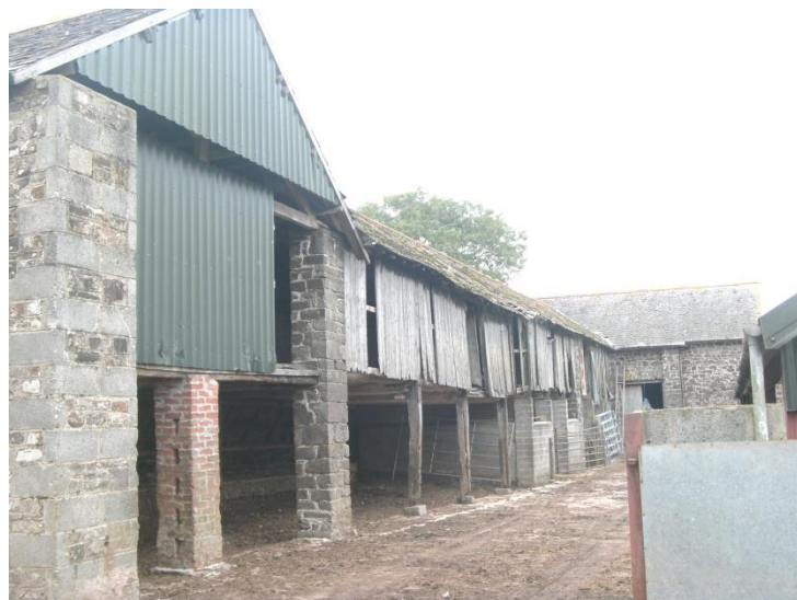
View of northern range; with modern supporting pillars at western end.
