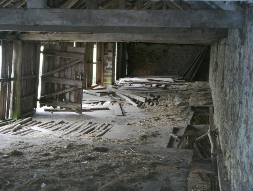
Upper floor of the long linhay east-west, fir pole flooring in evidence
