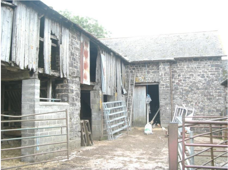
The linhay and granary before restoration
