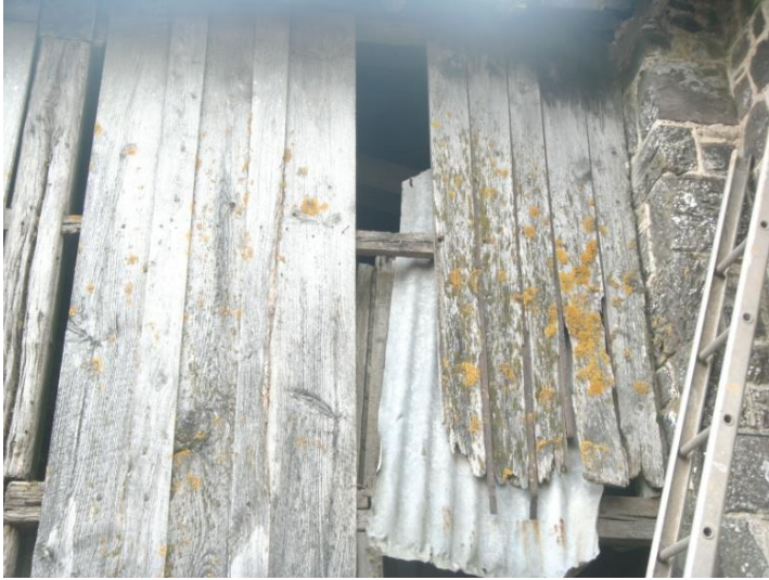
External boarding to the upper floor of the engine house; note metal strips between boarding
