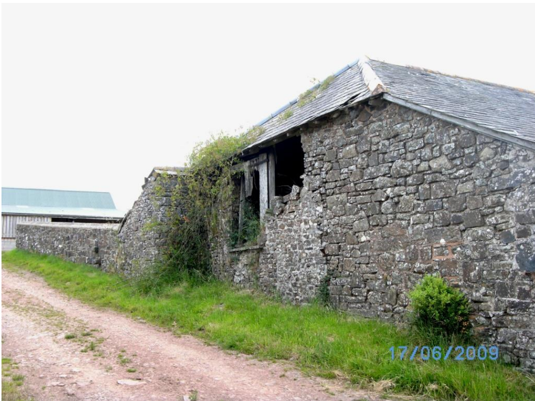
Western elevation of end of cider house (part of the old wall shown on tithe map?)
