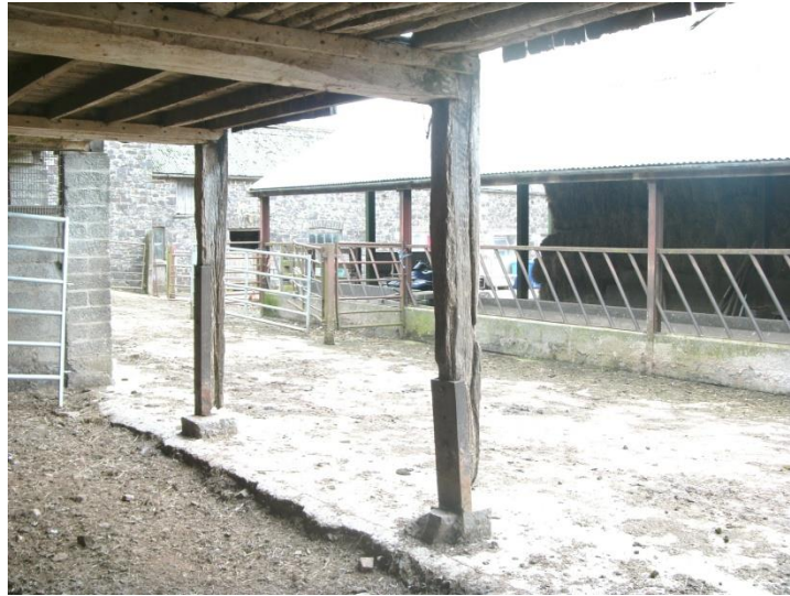
Supporting posts with metal strengthening. Modern barn in front
