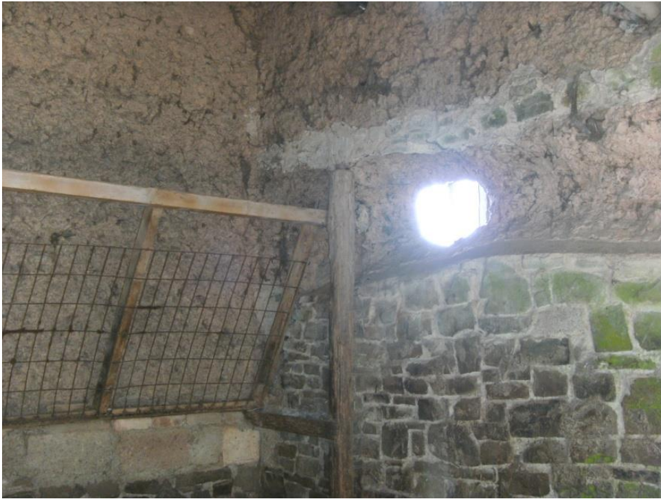
Hole through the cob in eastern end, presumably for wooden beam
