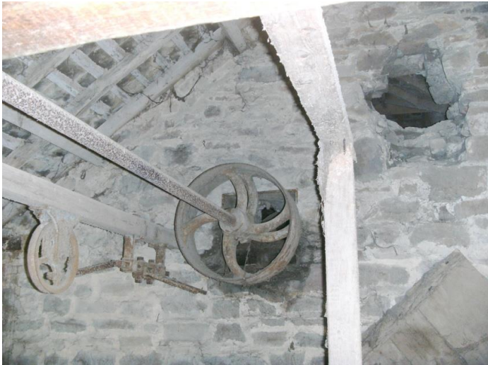
Remains of the pulley system from the upper linhay, into the granary
